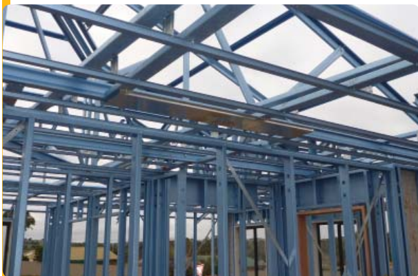
Additional bracing for the support of a garage panel lift door.
