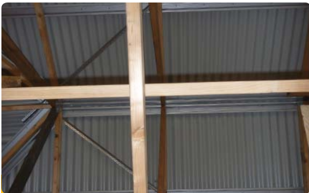
Distorted trusses
