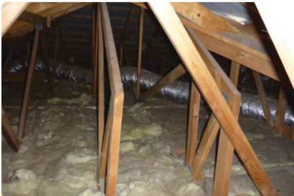
Unbraced trusses
