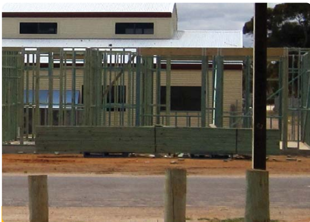
Trusses stored on a flat site
