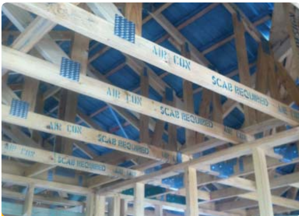
Trusses indicating location of proposed air conditioning unit.
