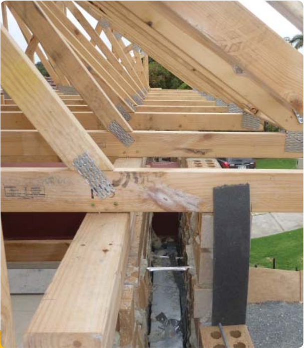
Cantilever correctly installed.
