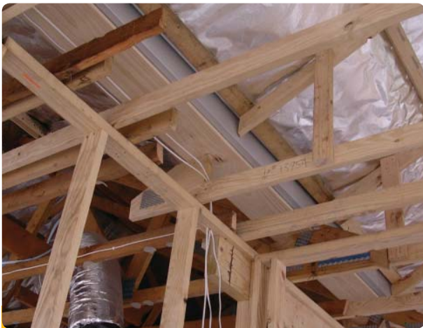
Modified roof trusses
