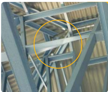
Damaged brace
