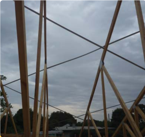
Steel brace installed to top of roof trusses
