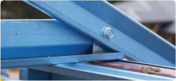
Typical tie down at the pitching point of a truss.
