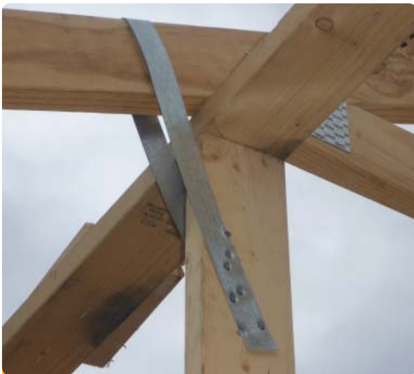
Typical strap tie downs at the pitching point of a truss.
