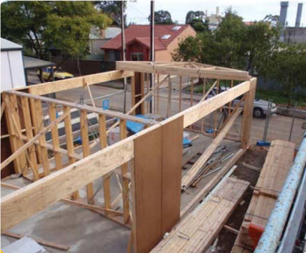
Trusses stored on top of wall frames
