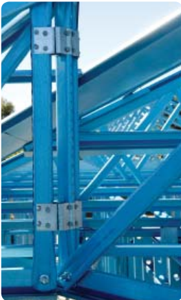
Typical tie down at the pitching point of a truss.
